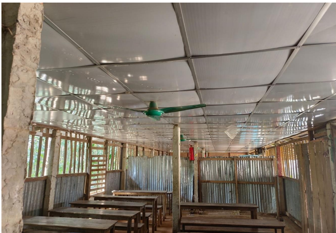
Picture 5: Host community school retrofitted with tin barrier and new roof
