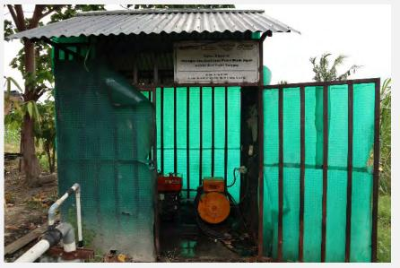
A water pump powered by diesel (in the middle)
