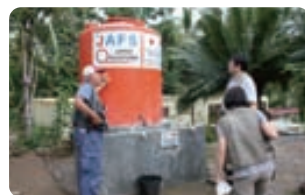
Emergency Assistance ① JAFS staff and experts monitoring a water station. ©JPF
