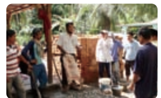
Emergency Assistance ② SNS staff providing technical training to the affected people during construction coaching tour. ©SNS
