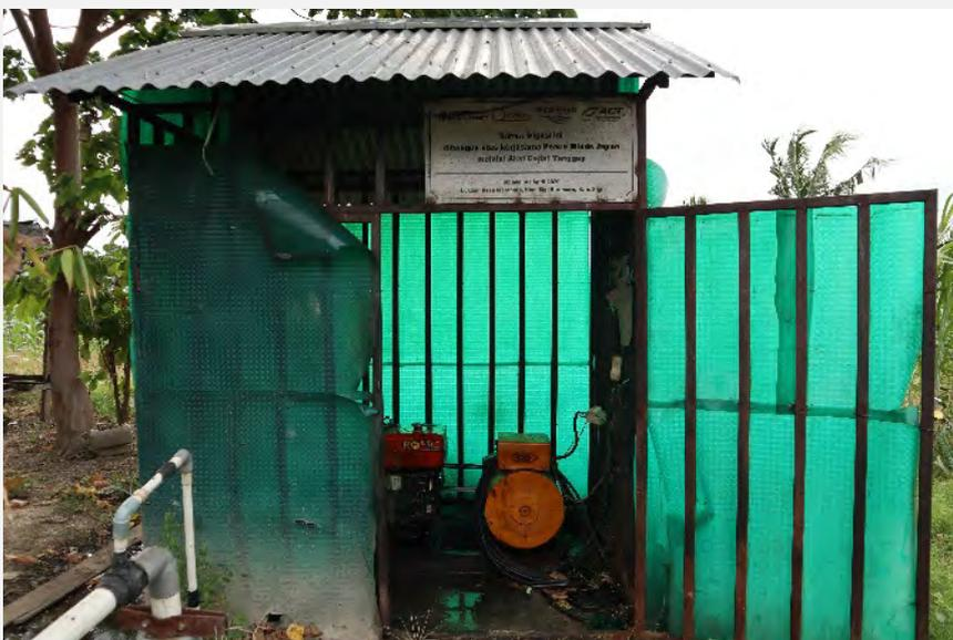
***A water pump powered by diesel***
